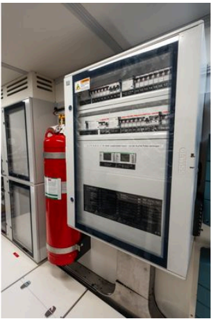
Electrical panel and fire extinguisher on 2024 Cranchi Sessantasette 67 yacht.
